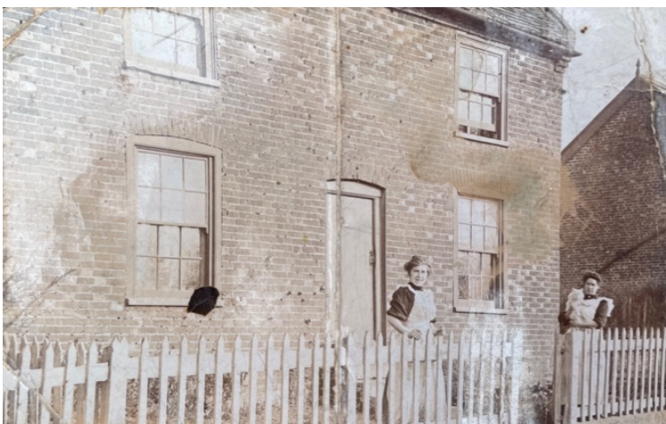
The cottage at Craggs' Farm
